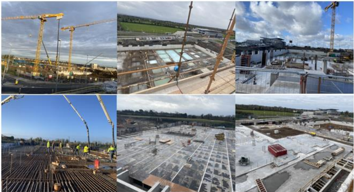
Figure 4: Basement Construction in Reinforced Concrete
