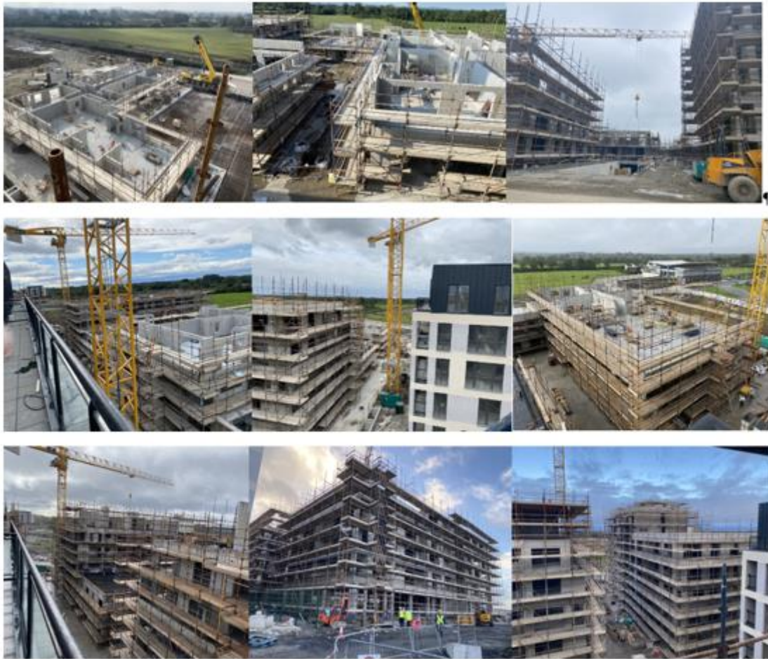
Figure 7: Apartment Block Construction in Precast Concrete
