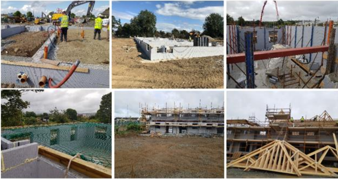
Figure 8: House Construction in ICF
