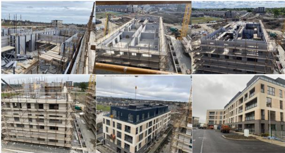
Figure 6: Apartment Block Construction in ICF
